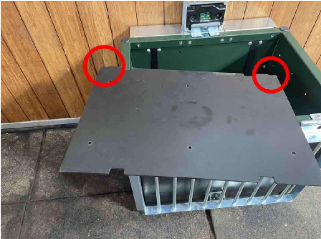
[ ] Secure the feed floor with six M6x20 flange bolts.
