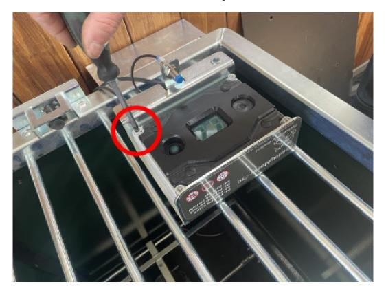
[ ] Place the front of the controller housing next to the controller. Feed the motor cable through the strain relief into the controller housing. Do not tighten it yet.
