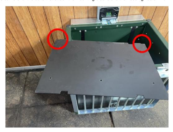
[ ] Secure the feed floor with six M6x20 flange bolts.
